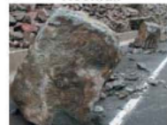
Photo courtesy Colorado Department of Transportation (CDOT)
