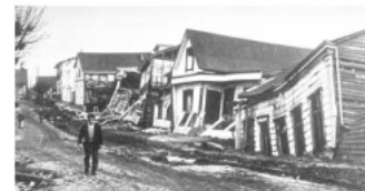
Damage Caused by the 1960 Chile Earthquake
